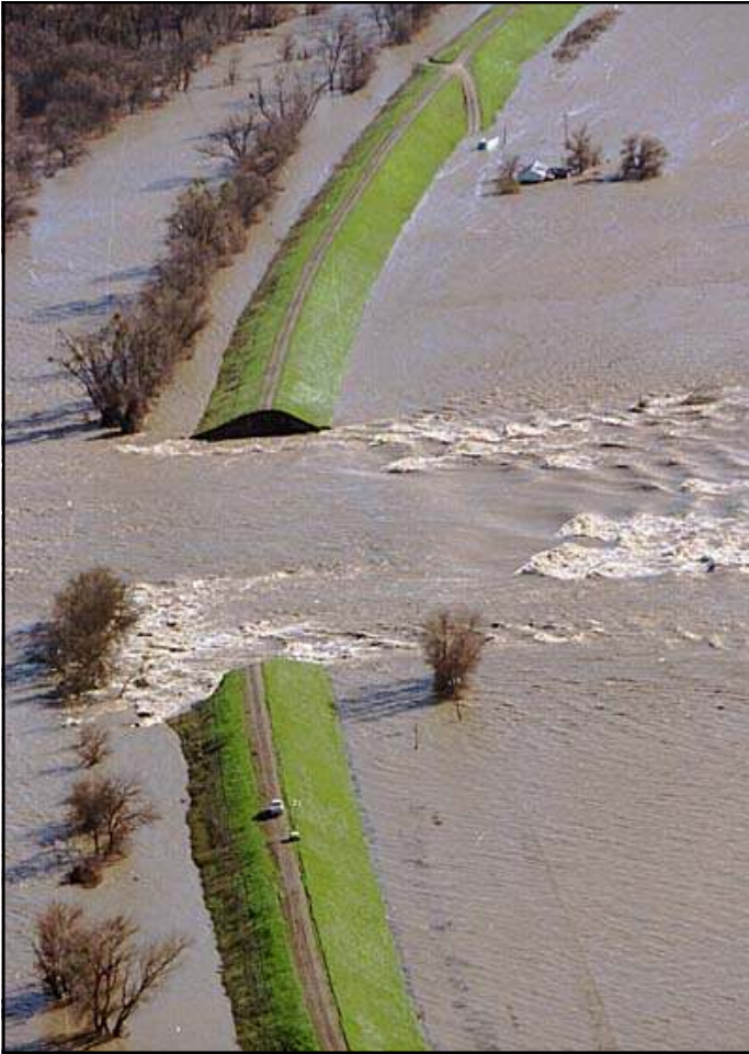
After a temporary obstacle, the Mississippi once again has its way in 1993. The Great Flood cost Missouri taxpayers over $14 billion. In the years since then, more flood plain development has occurred in Missouri than in any other time in history.
